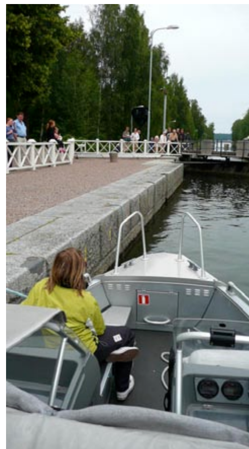
Going through the Vääksy channel from Vesijärvi to Päijänne. The water level in Vesijärvi is some 3 meters higher than in Päijänne.
